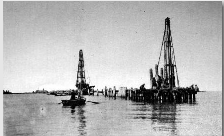
The beating of the pillars by the help of the steam drop hammer equipped with a 500 - 1,000 kg ram.
