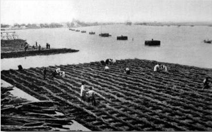
The dams' prolongation with fascine mattress launched by floating and bound up with wire (1921 – 1930)
