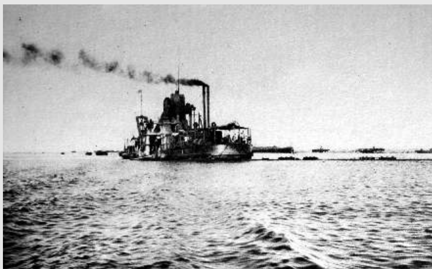
Sir Charles-Hartley drag with brackets (Built in 1891, 250 PH, 37.79 m length, 8.53 m breadth, 3.95 m draught, 313,57 t brute tone)
