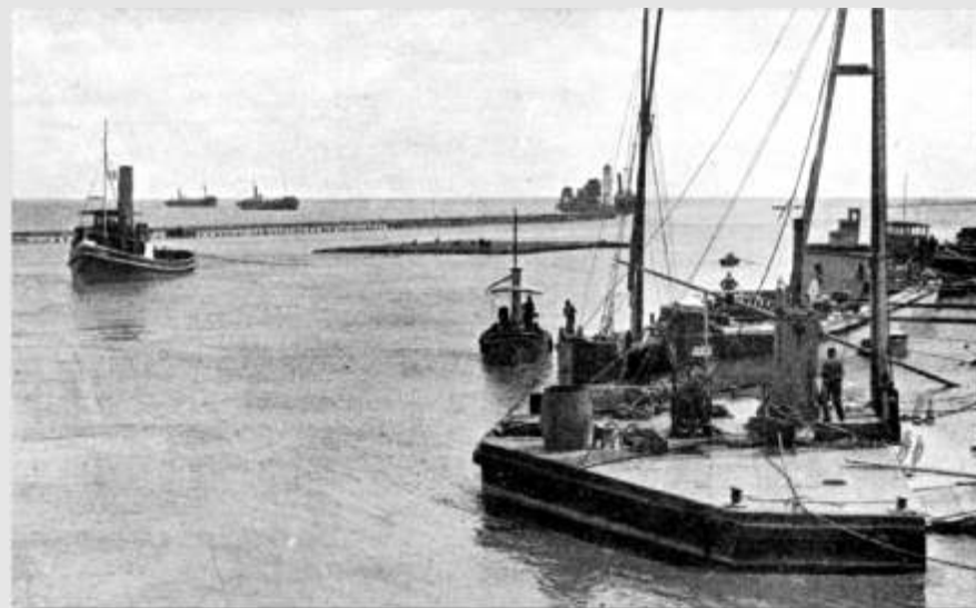
Ismail tug boat (Built in 1919, 500 PH, 28.80 m length, 6.40 m breadth, 2.60 m draught, 145.02 t brute tone, 10 running-knot speed)
