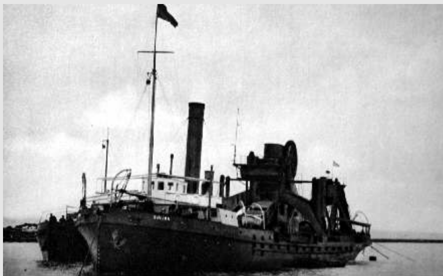
Sulina drag with brackets (Built in 1923, 950 PH, 67 m length, 12.80 m breadth, 5.33 m draught, 1,164.75 t brute tone, 420 mc capacity, 8 running-knot speed)
